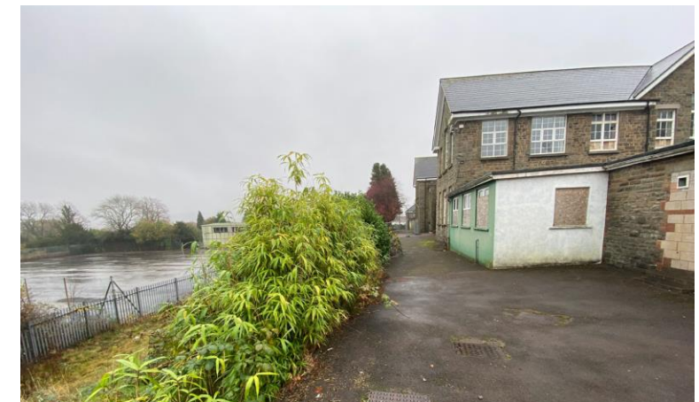
6 View looking East onto Tennis Courts
