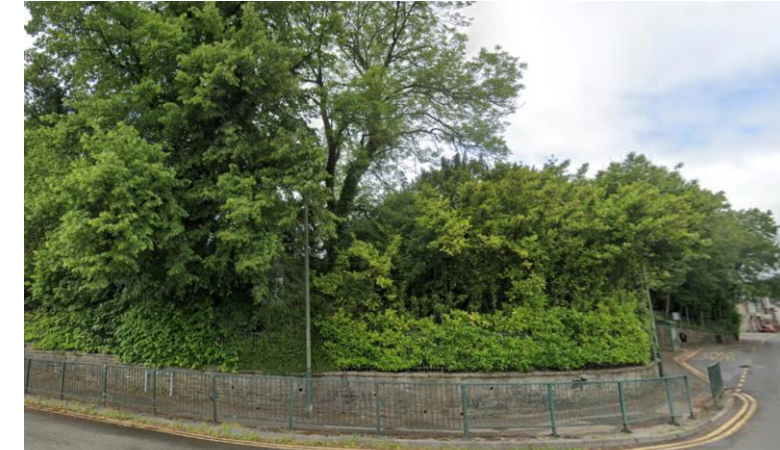
3 Mature trees and retaining wall to NE Boundary
