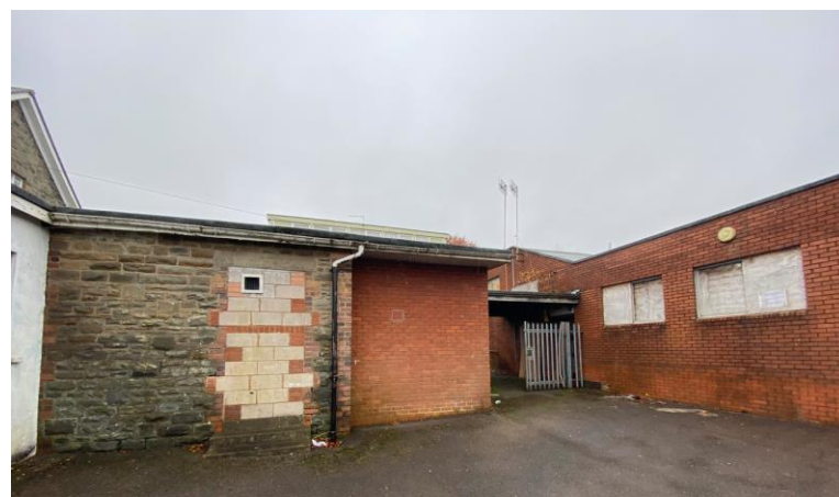
7 Covered walkway link to existing Red Brick building
