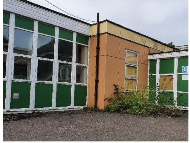
Photo 90: Lifted Cladding
