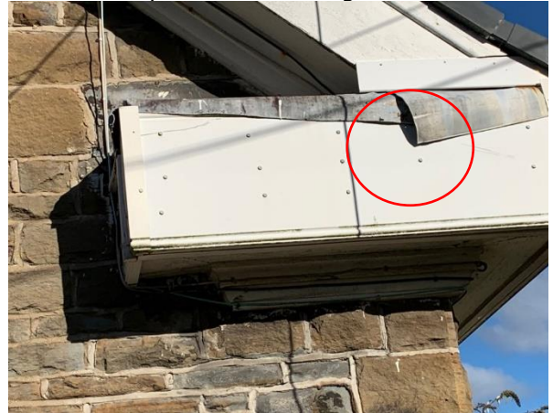
Photo 68: Gaps in Lead Flashing.
