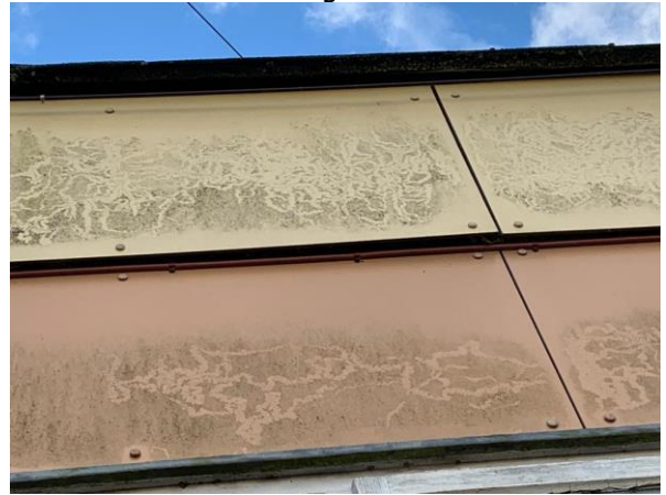
Photo 90: Lifted Cladding
