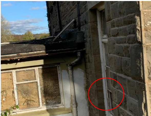
Photo 67: Gap Between Wall and Soffit.
