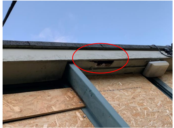
Photo 114: B12 Gap in Soffit Box.
