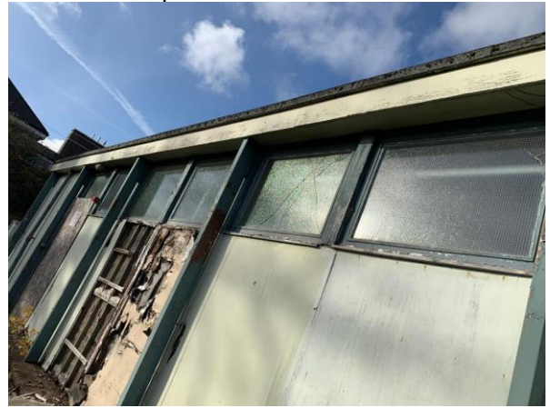
Photo 114: B12 Gap in Soffit Box.
