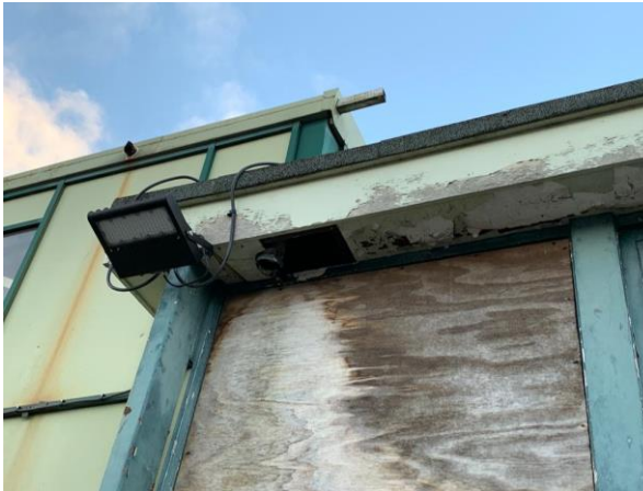
Photo 113: B12 Security Light and Gap in Soffit Box.
