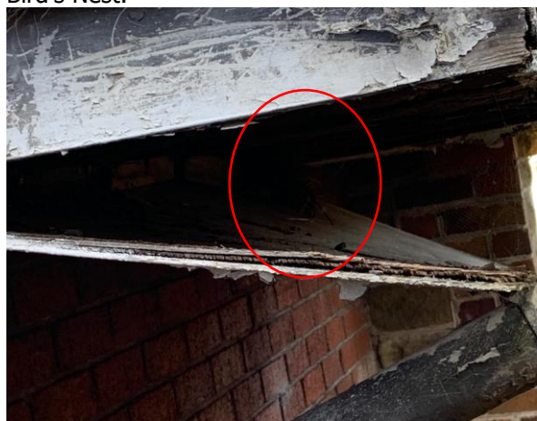
Photo 77: B1 Broken Soffit with Large gap and Bird's Nest.
