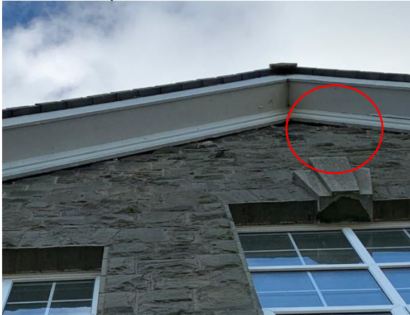
Photo 67: Gap Between Wall and Soffit.
