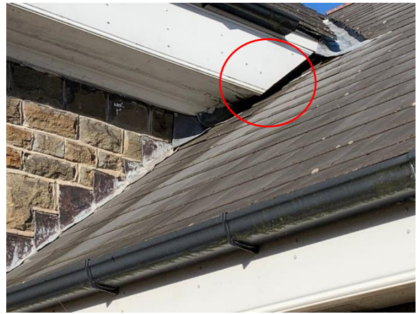
Photo 68: Gaps in Lead Flashing.
