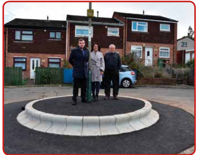
Completed roundabout in Churchill Park, Caerphilly.
