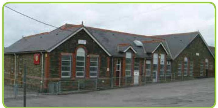
The former school
