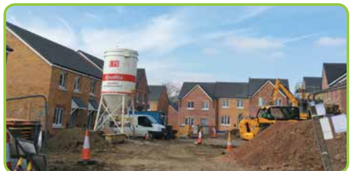
The site under construction
