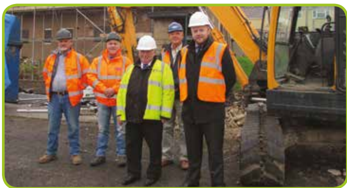
Cllr David Poole (Deputy Leader of the council & Cabinet Member for Housing) with ward member Cllr Carl Cuss and Cuddy Demolition
