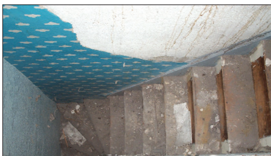
View of stairs from landing
