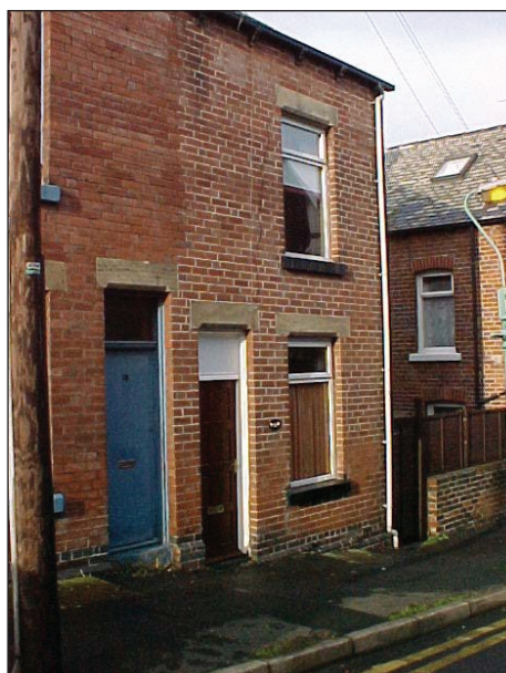
Narrow frontage house Dwelling: pre-1920 mid-terraced
