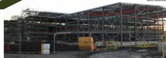
Progress at the Islwyn High School site.
