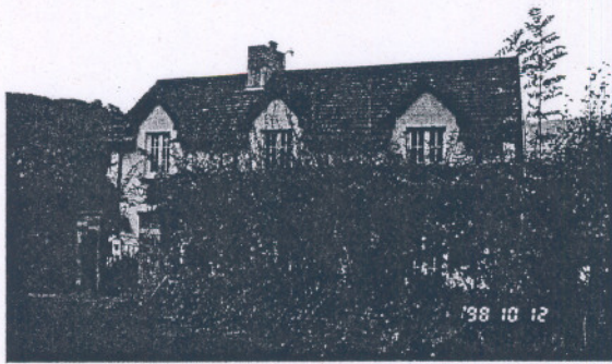
5. Traditional windows and openings.
