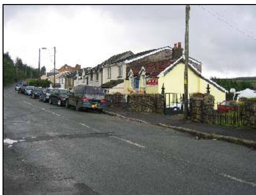
Photo 3 – existing housing along Merthyr Road
