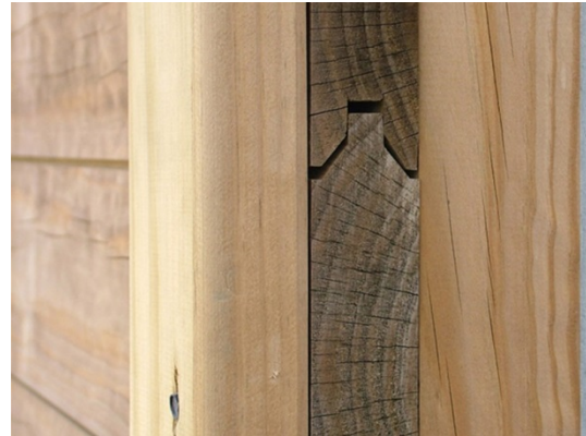
Figure ESA13.2 Detail of Acoustic Fence Boarding
