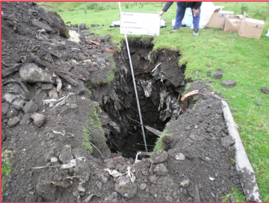
Above:- TP01 spoil
