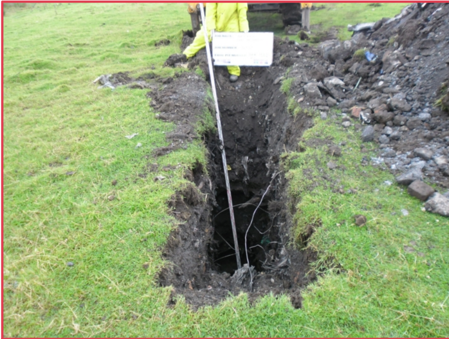
Above:- TP04 spoil
