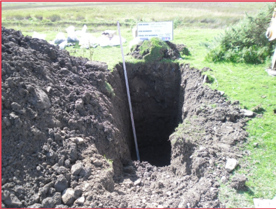
Above:- TP12 spoil
