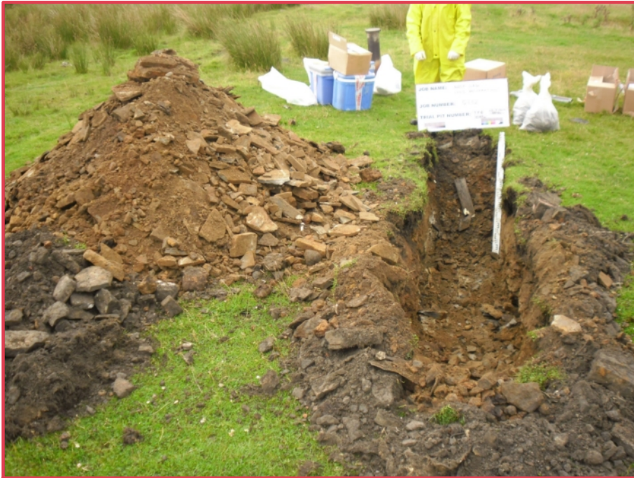
Above:- TP06 spoil
