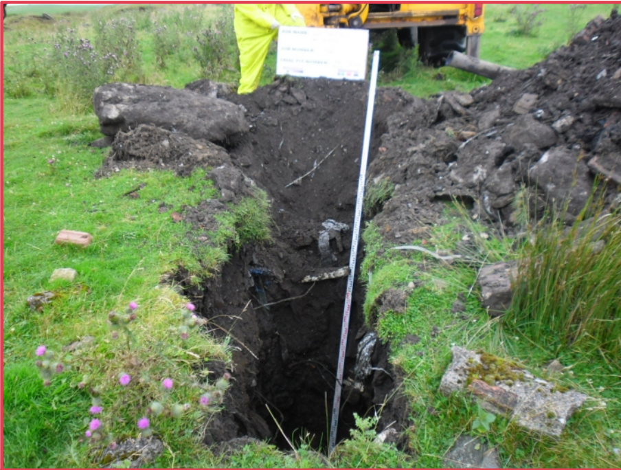
Above:- TP08 spoil
