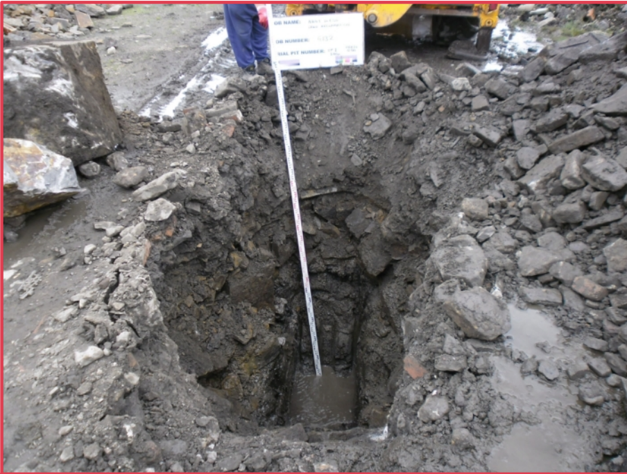
Above:- TP11 spoil
