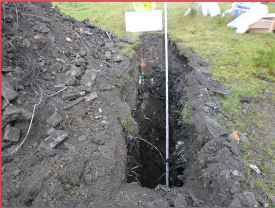
Above:- TP05 spoil
