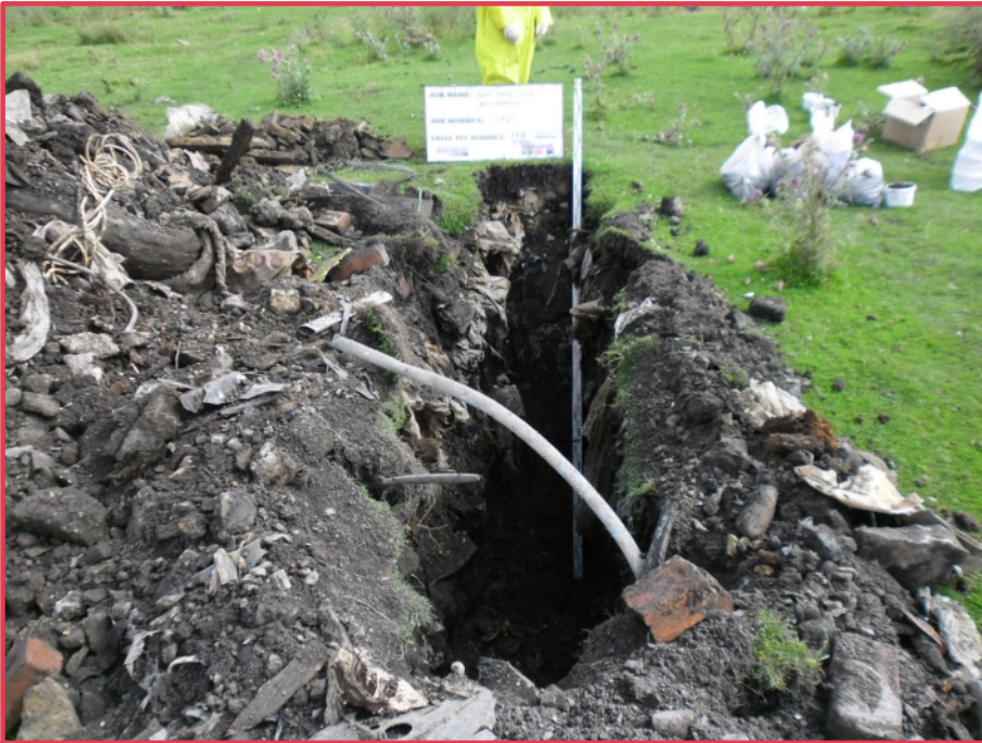
Above:- TP07 spoil
