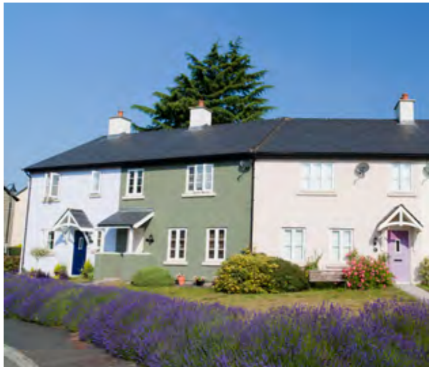
Terraced housing turning a corner
