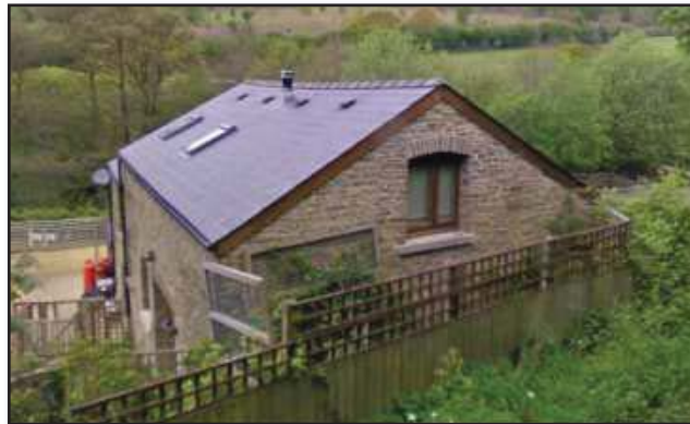
Discreet venting tiles and flue on the least visible elevation
