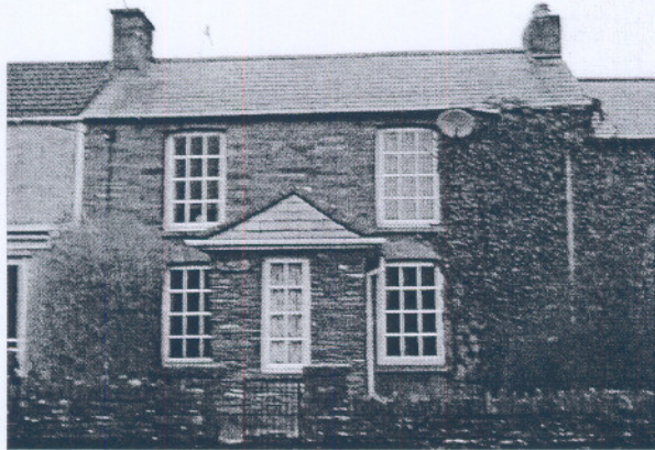
Photograph 13: An Original Porch on High Street, Nelson
