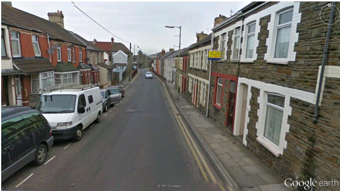
Figure 3-5 White Street- “street canyon”
