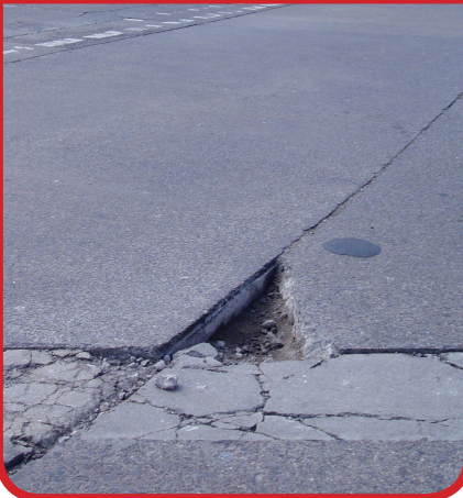
Actionable pothole
