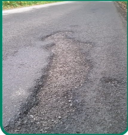
Non-actionable pothole
