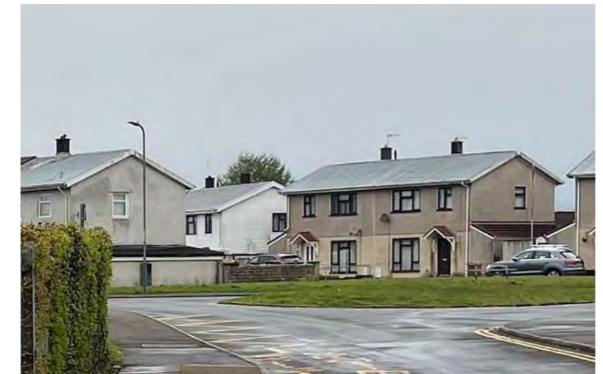
Figure 5 - BISF Housing to West of Site
