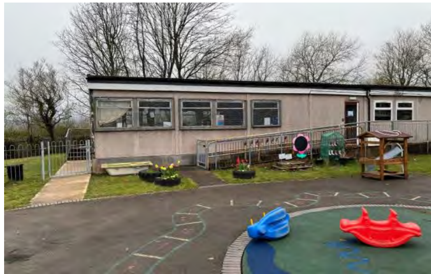
Figure 9 - Existing prefabricated building for demolition
