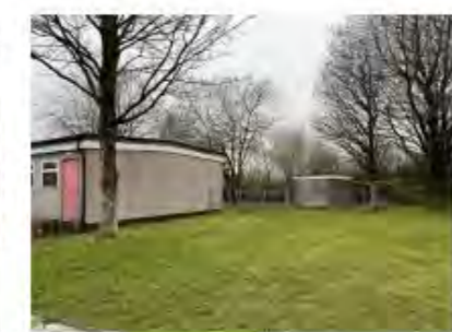
Buildings 1381 (on left) & 1793 (on right)
