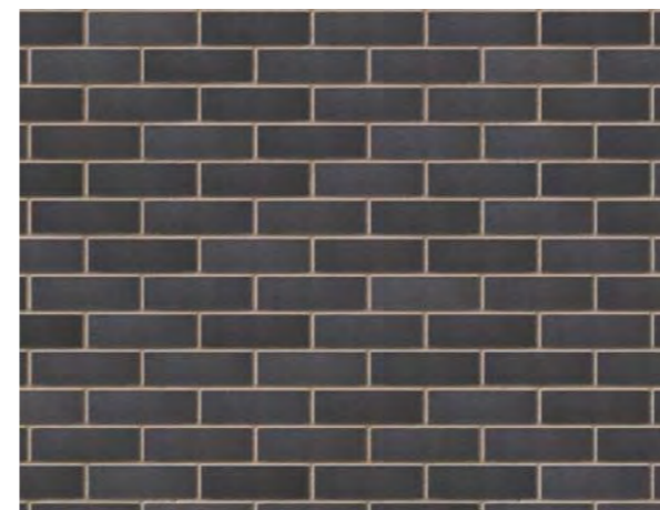
Below DPC brickwork - Staffordshire Blue engineering brick laid half lap stretcher bond
