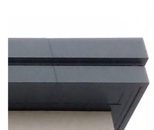
Soffits and Facias to Extension - Aluminium - Anthracite (RAL 7016), Aluminium rainwater goods (RAL 7016)
