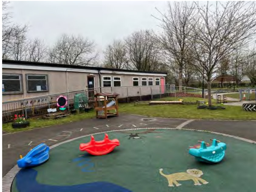
Figure 8 - Existing prefabricated building for demolition
