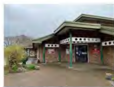
School Entrance - Building 329
