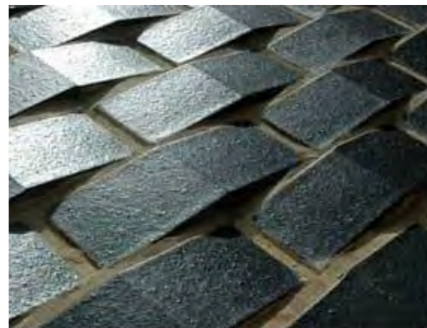
Feature brickwork - Istock Umbra sawtooth laid half lap stretcher bond - Staffordshire Slate Blue smooth
