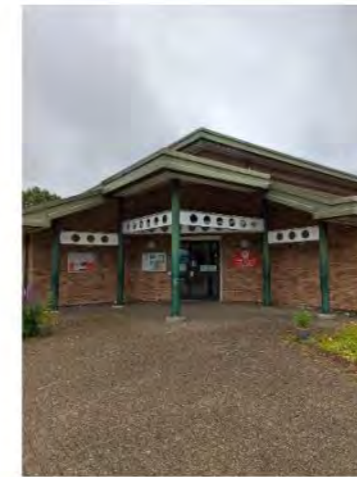
Figure 17 - Main entrance to the school at the north western corner of the building.
