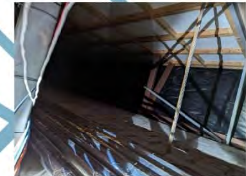
Figure 20 - Visible loft space at the west of the building.
