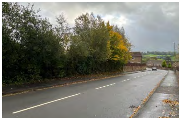
Figure 22 - External view of site from the South
