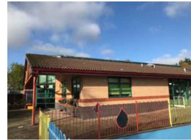
South Western corner of existing building
