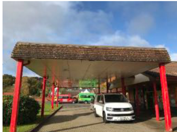
Existing Entrance & Covered Drop-off
